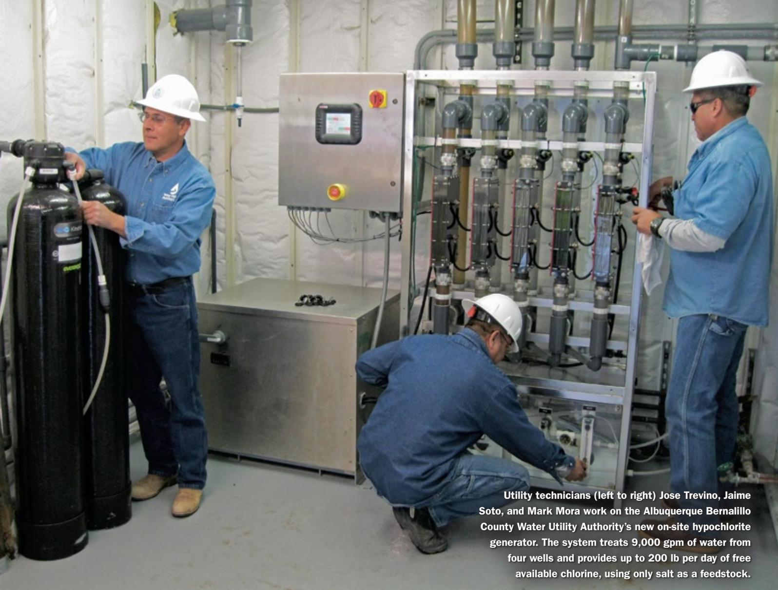
Utility technicians (left to right) Jose Trevino, Jaime Soto, and Mark Mora work on the Albuquerque Bernalillo County Water Utility Authority's new on-site hypochlorite generator. The system treats 9,000 gpm of water from four wells and provides up to 200 lb per day of free available chlorine, using only salt as a feedstock.
